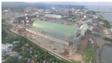
Photo 1: Installation is currently underway on the Limay II Project (Photo SCHADE).
