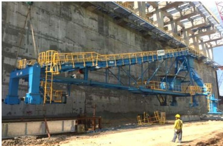
Photo 2: The Tripper Car was completely pre-assembled and lifted onto the rails with a crane. (Photo SCHADE)
